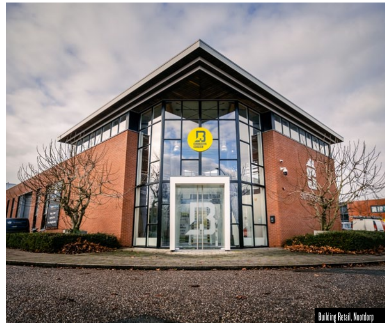
Building Retail, Noordorp
