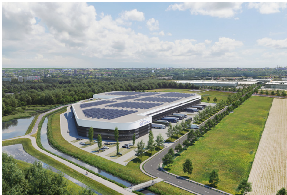
Cold storage centrum Ridderkerk
